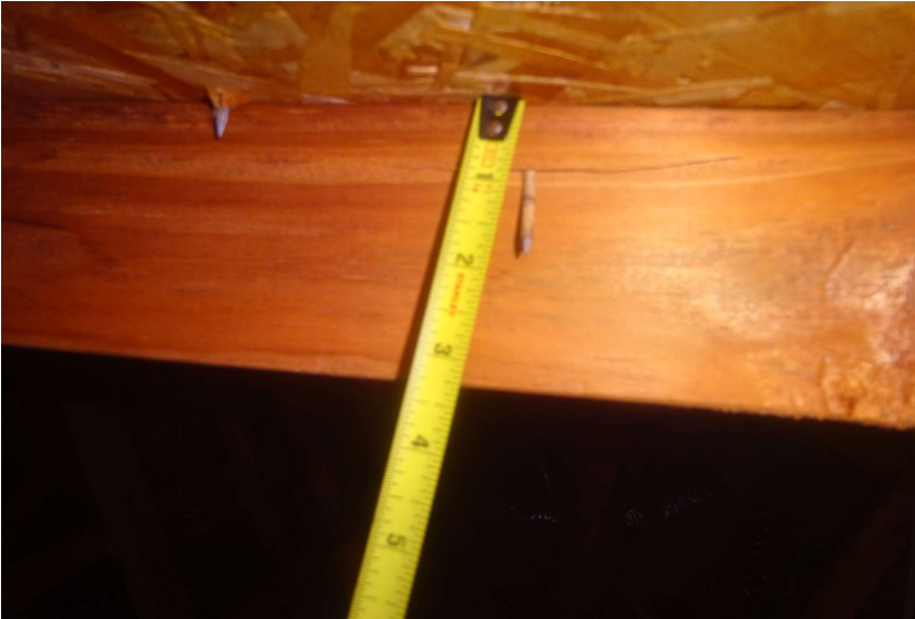
8d nails verified
